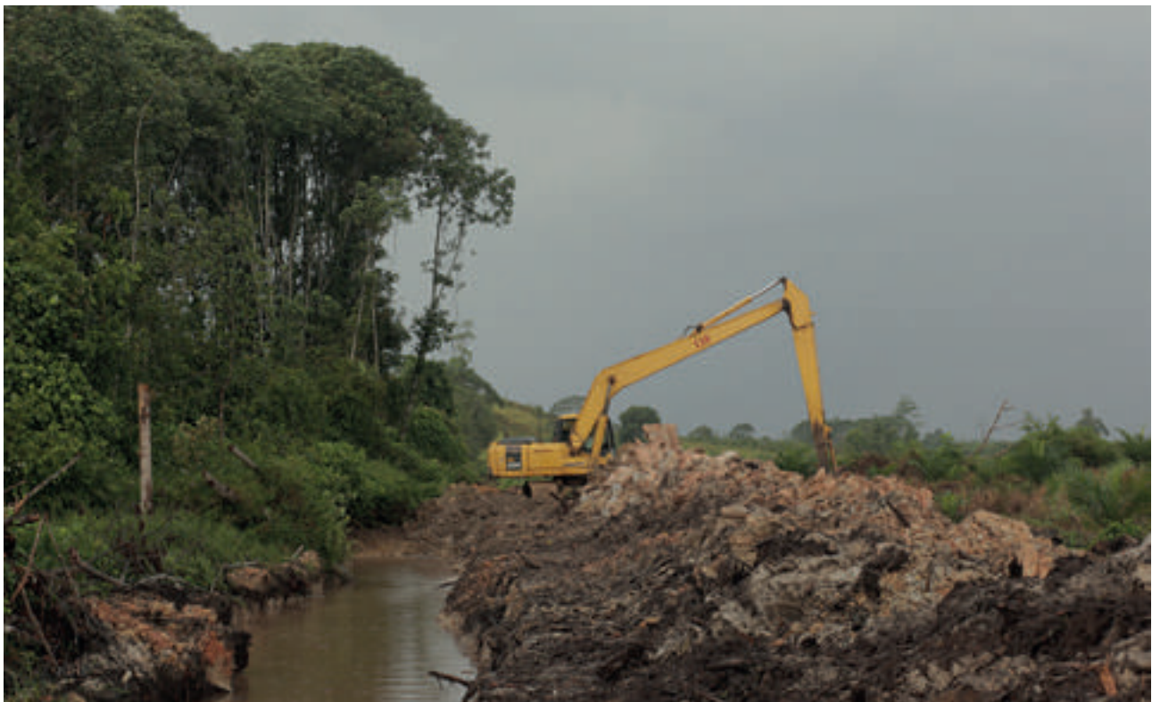
Digging of drainage canal next to natural forest in LSM plantation.
